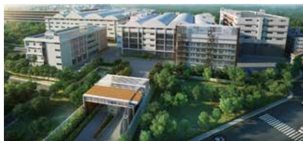
Srijan Industrial Logistic Park on NH 6
